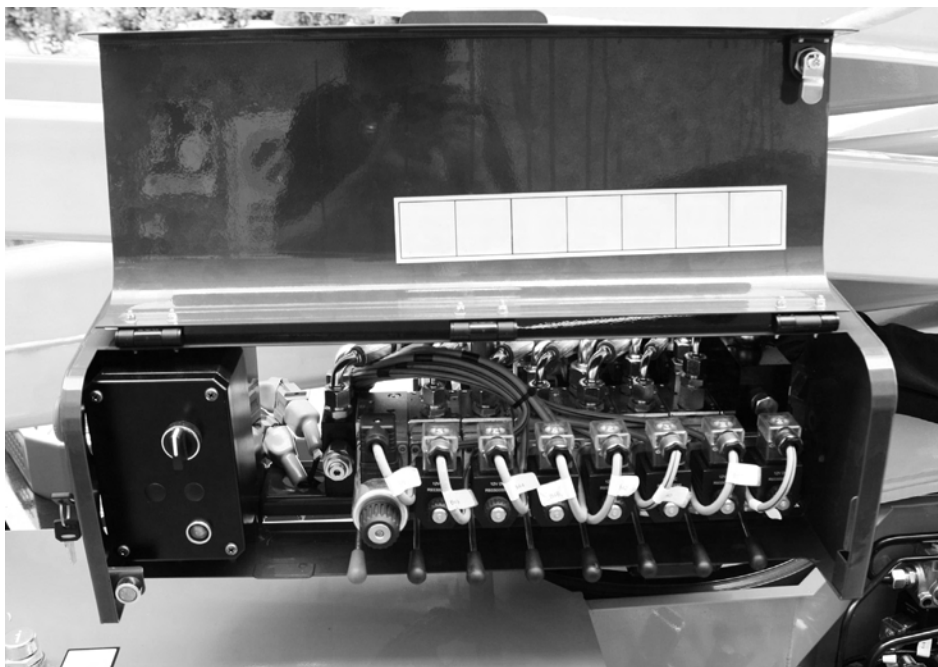
Fig. 79 Controls distributor of aerial part
